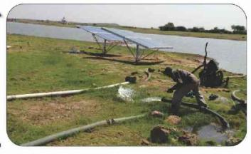
Irrigation pumps such as submersible, surface or deep well can also be coupled with drip irrigation systems to enhance the returns from this configuration.
