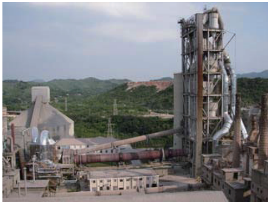
Waste heat recovery power plant for cement plant (Conch Cement in China)
