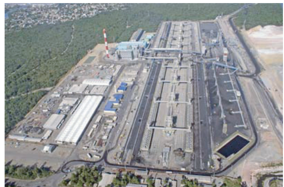
Waste heat recovery power generation equipment for coke oven (SOL CST in Brazil)
