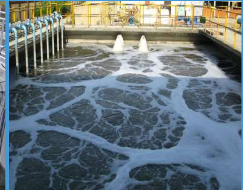
SEWAG TREATMENT PLANT (EA)
