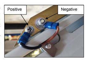
Fix the charging station with the limit assembly onto the steel profile in the upper and lower landing. Fine adjust limit switches S27 and S28 if necessary with the slot hole under the carriage covers.
