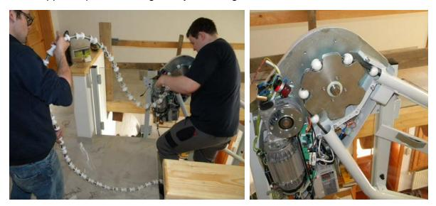
• Enter the lower rope into the over speed governor tube section. It might be necessary to release the tension spring in order to facilitate entry of the rope into the safety gear tube section. This spring later should be set to the same tension again after the rope is installed!
