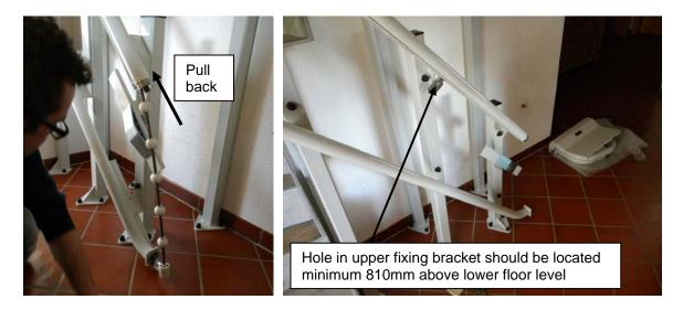
• Add the current collector into the upper tube next to the fixing bracket. Make sure the spring between the current collector and the upper fixing bracket is securely attached to the current collector. This spring is responsible to make the electrical contact between the tension cable and the platform control board.
