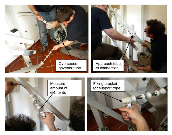
It is important that there are not too many support elements on the support rope as then it is not possible to tension the cable. A gap between the last support element and the fixing bracket of the support rope is ideal. This gap depends on the length of the rail and number of curves and is later reduced when the rope is tensioned! Below a table that shows approximate gap length based on rail length.
