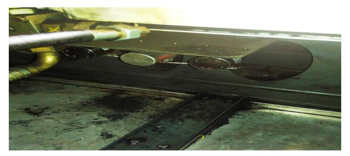
FirePro Aerosol generators installed in the lower section of the crane's engine room.
