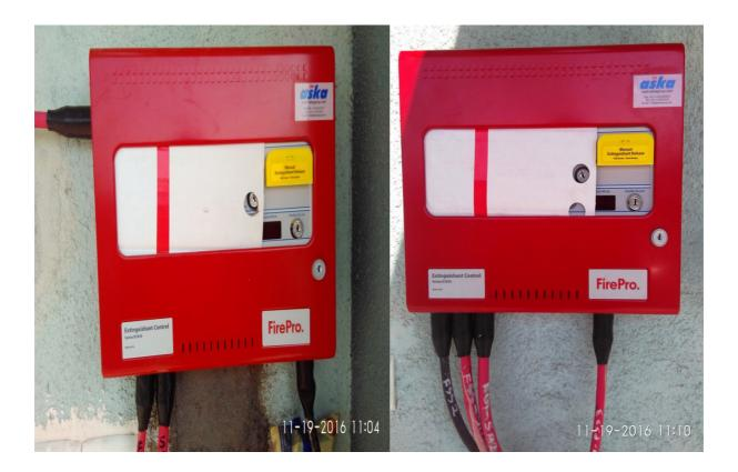
We have provided the Aerosol based fire suppression system for 2 rooms at Reliance Gas Pipe Line project. 1. Battery room. 2. Electrical panel room.
